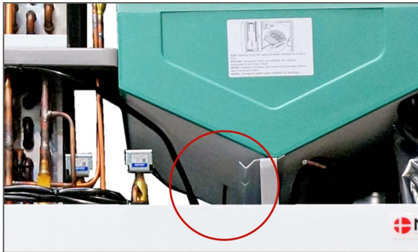
1. Remove the T4 sensor in the heat exchanger.
