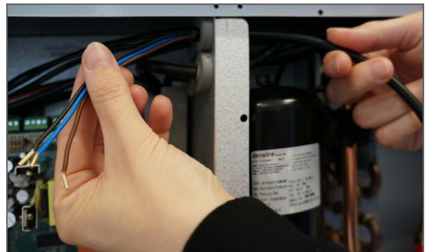
6. Run the wire from the CO 2 sensor through the cable grommet to the automation. Wire is subsequently tied up with cable strips.
